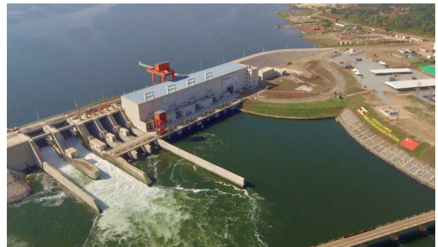
乌干达伊辛巴水电站项目 (EPC, 183.2MW) Isimba Hydro Power Plant & Isimba-Bujagali Interconnection Project, Uganda (EPC, 183MW)
